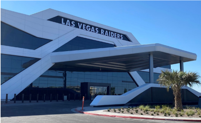
Las Vegas Raiders Headquarters & Practice Facility
